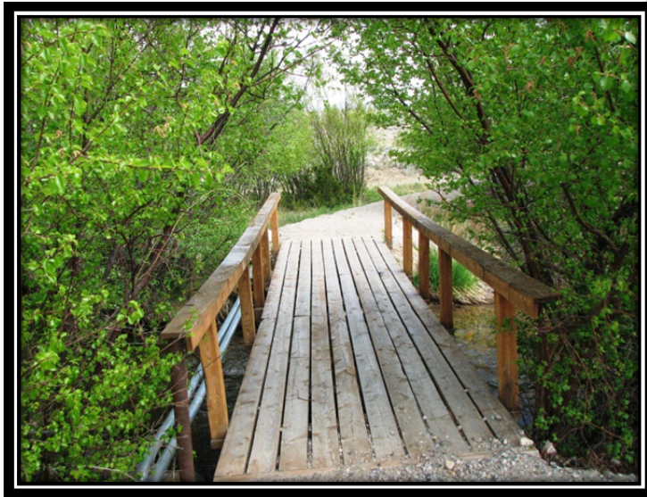
Bridge over Little Rock Creek
